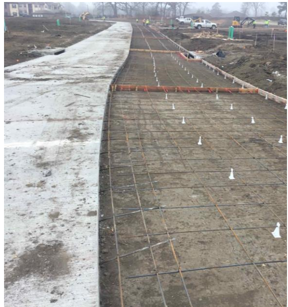
Installation of concrete roadway
