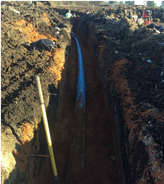
Installation of waterline
