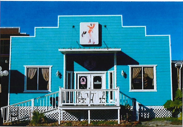
EXISTING REAR FACADE
