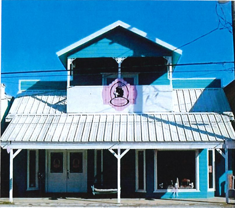
EXISTING FRONT FACADE
