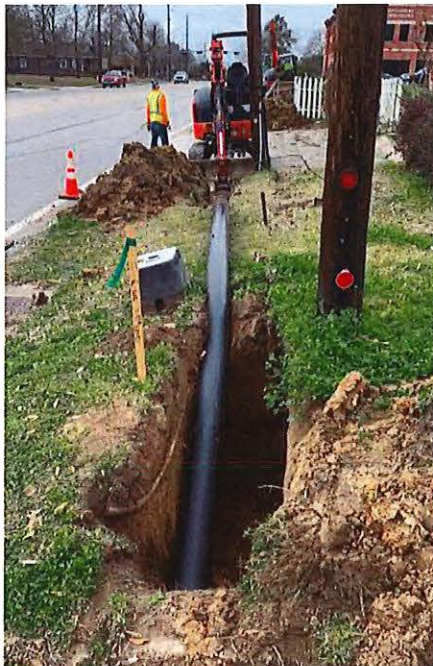
Temporary waterline along SH-105
