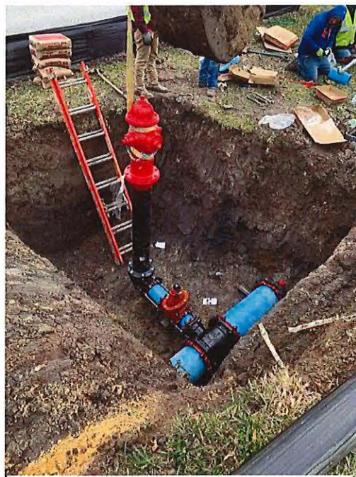
Flushing valve installation on SH-105
