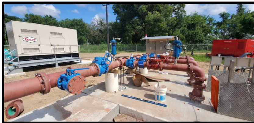
Lift Station Site
