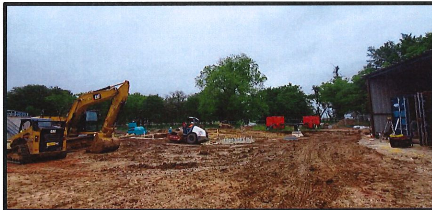
Lift Station Site
