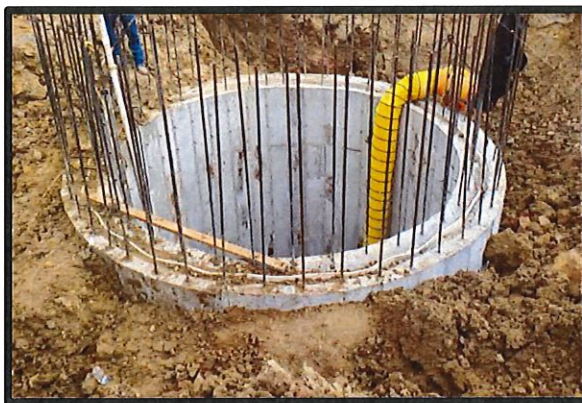
Lift Station No. 1 Wet Well
