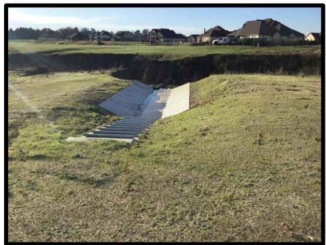
Additional slope paving
