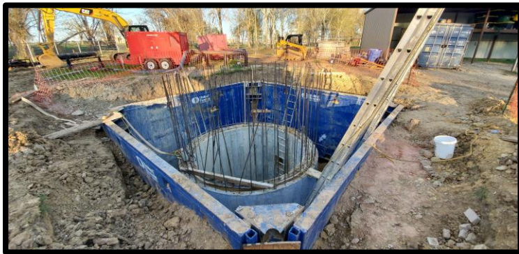
Lift Station No. 1 Wet Well
