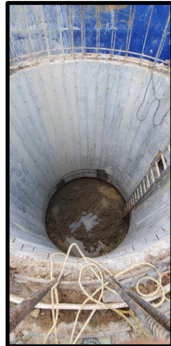
Lift Station No. 1 Wet Well
