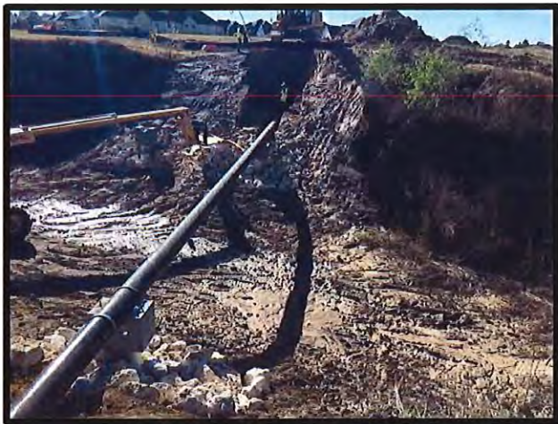
Waterline installed in casing across piles
