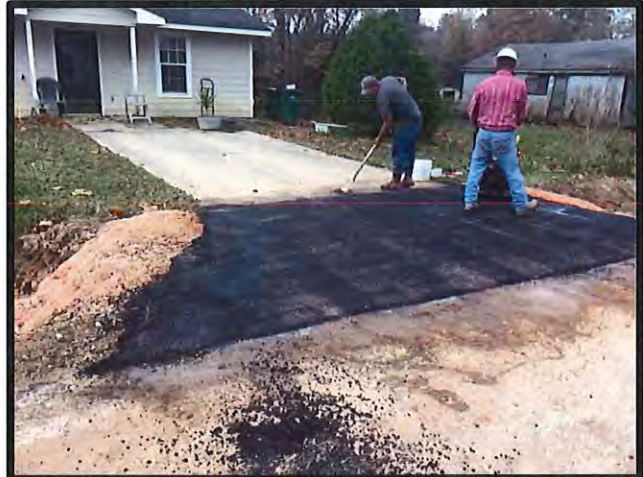
Driveway repair along Baja Road
