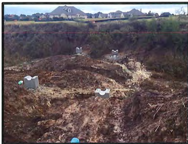
Pile caps complete and in place
