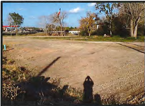
Lift Station No. 1, demolished and backfilled
