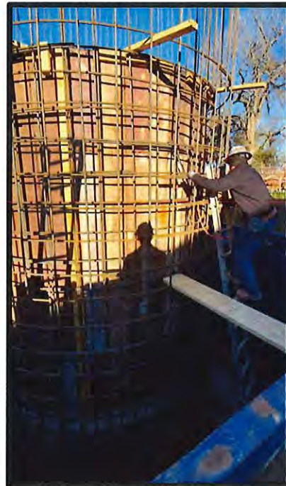
Rebar for new Lift Station No. 1
