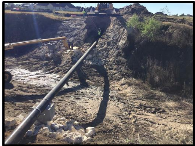
Waterline installed in casing across piles
