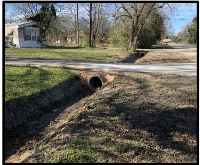
Ditch regrading & new culvert along MLK Drive
