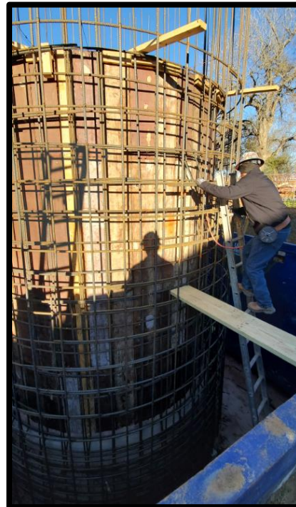
Rebar for new Lift Station No. 1
