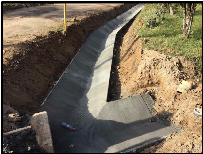
Roadside ditch along MLK Drive
