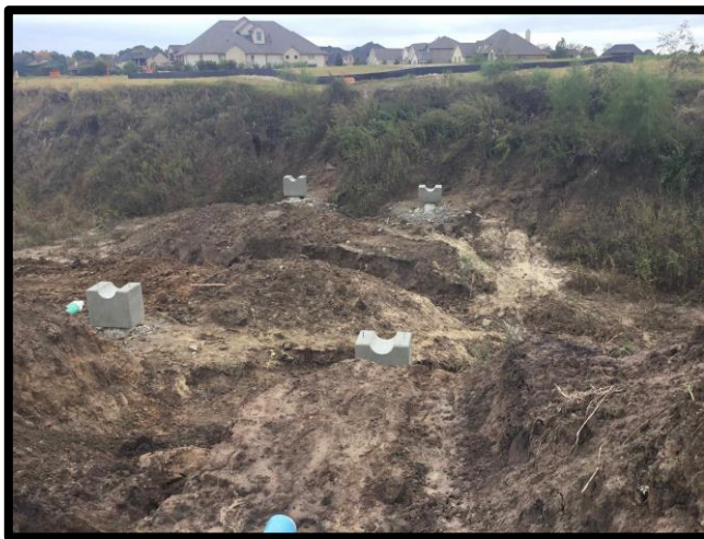
Pile caps complete and in place
