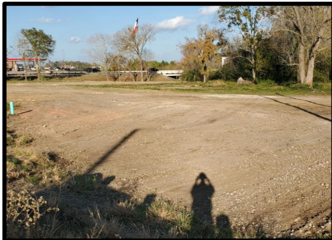
Lift Station No. 1, demolished and backfilled
