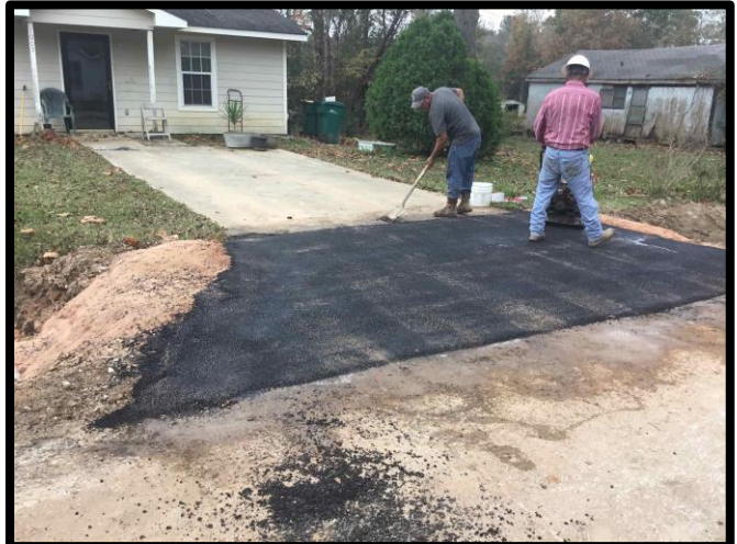
Driveway repair along Baja Road
