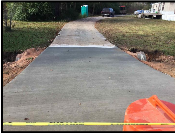
New culvert & driveway repair along MLK Drive
