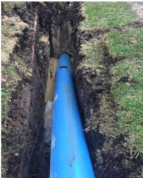
Trenchless construction on Pond St.
