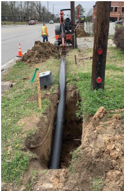
Temporary waterline along SH-105
