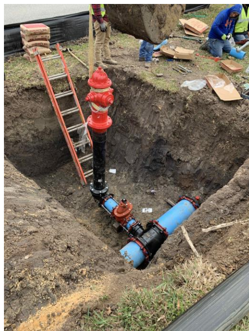
Flushing valve installation on SH-105
