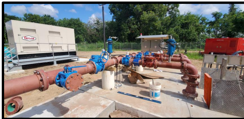
Lift Station Site
