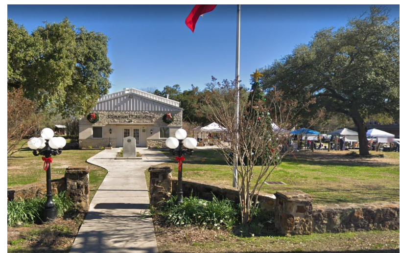
Figure 7.4 Montgomery Community Building
