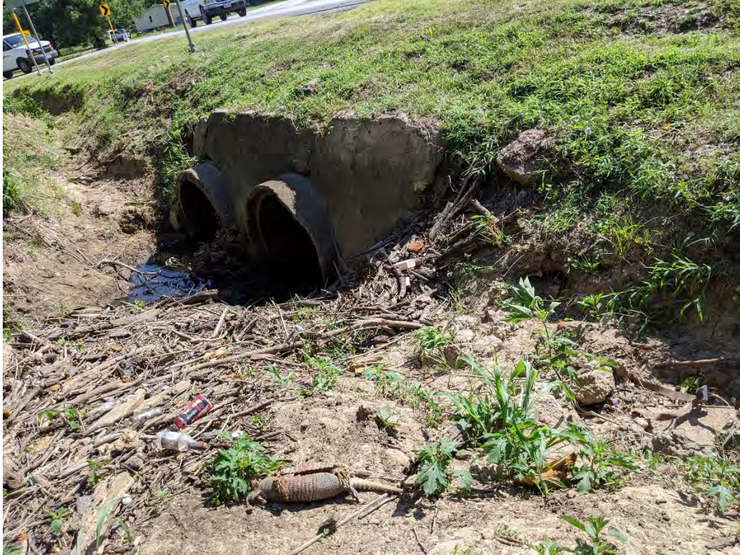
Upstream side of 2-54" RCPs at FM 149
