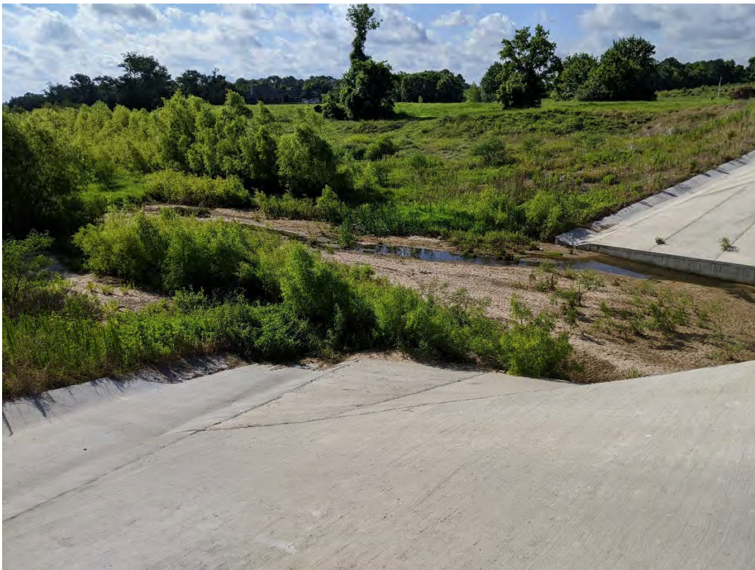
Downstream side of Buffalo Springs Drive, facing downstream
