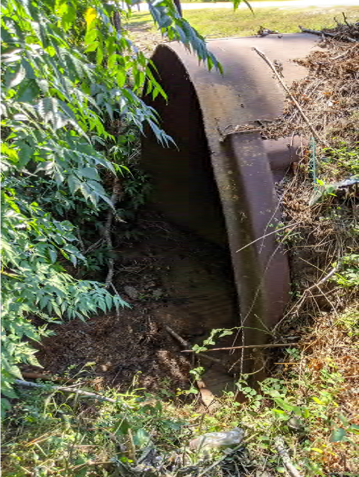
Upstream side of 108” steel pipe at MLK Drive
