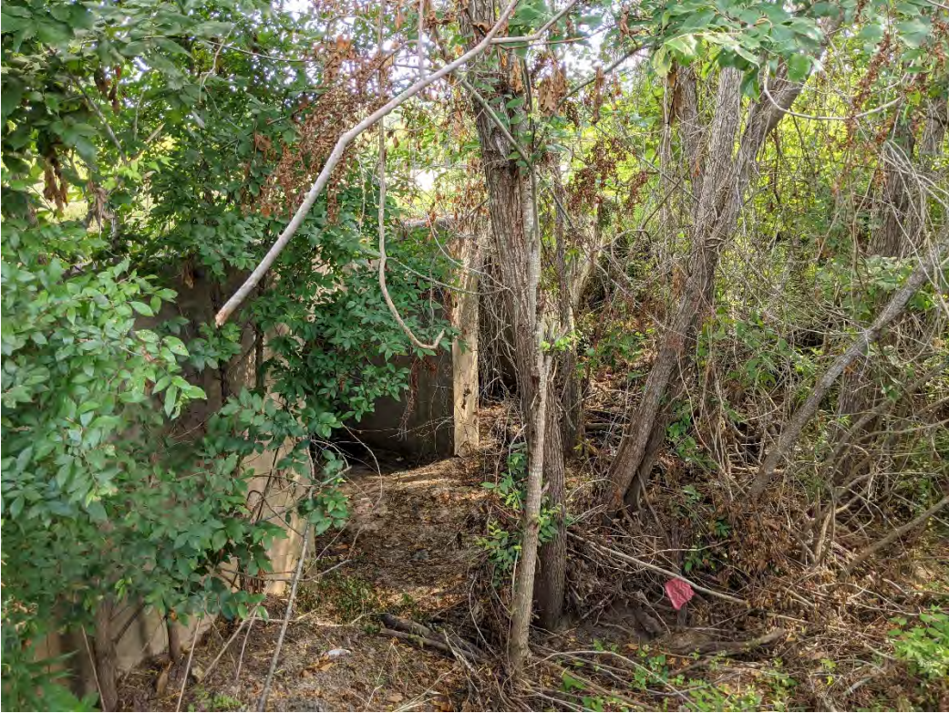
Downstream side of Plez Morgan, facing upstream
