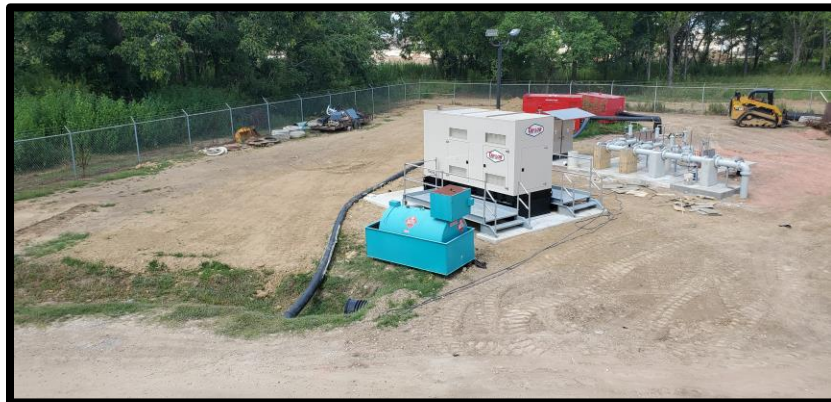
Lift Station Site
