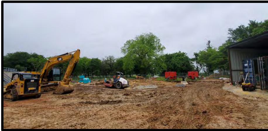
Lift Station Site
