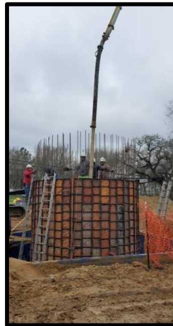
Lift Station No. 1 Wet Well
