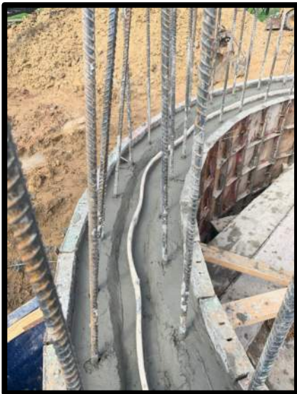
Lift Station No. 1 Wet Well
