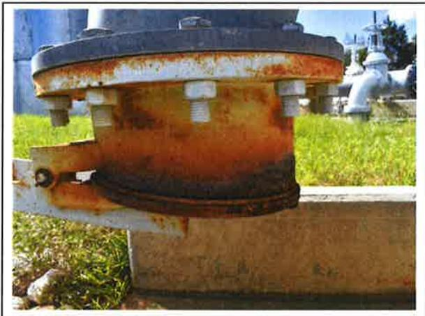
Findings: The protective coating on the overflow drain is failing.
