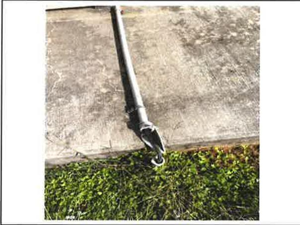
Findings: The conduit for generator ground is broken.
