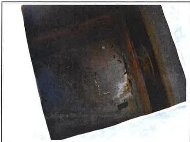
Findings: Corrosion and delamination around edges of overflow box.
