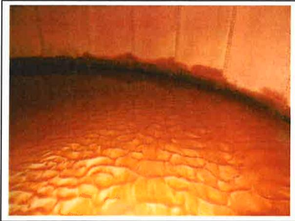
Findings: Sand is accumulating inside the tank.
