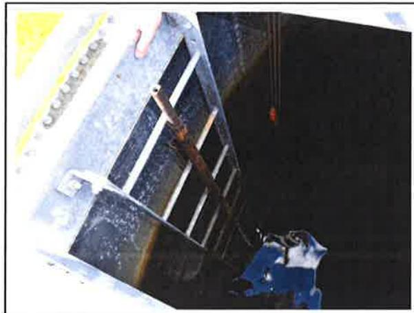
Findings: Corrosion on safety climbing feature on ladder.
