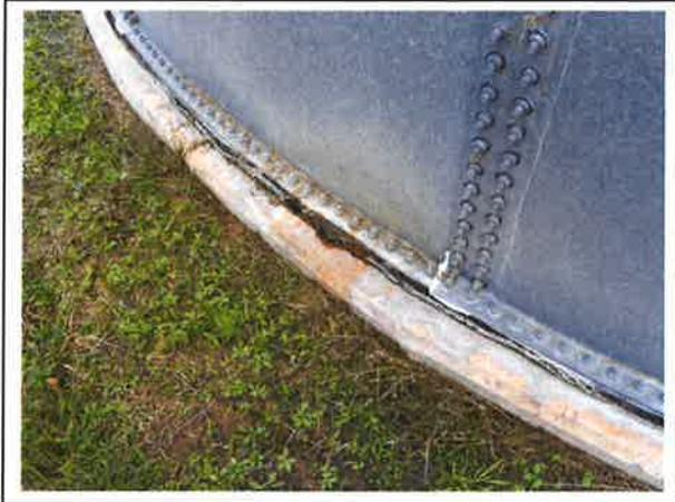
Findings: The foundation is wet and stained around isolated areas of the foundation.
