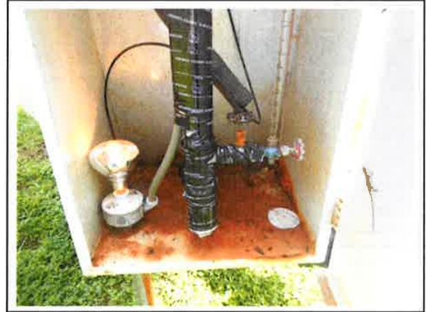
Findings: The tank cabinet and outer shell is delaminating inside the tank cabinet.
