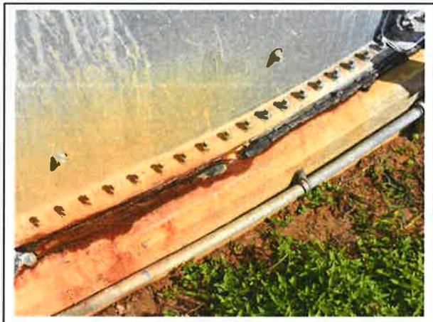
Findings: The foundation sealant is failing in isolated areas.
