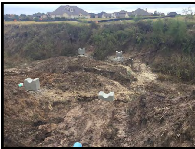
Pile caps complete and in place
