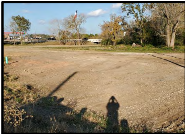
Lift Station No. 1, demolished and backfilled
