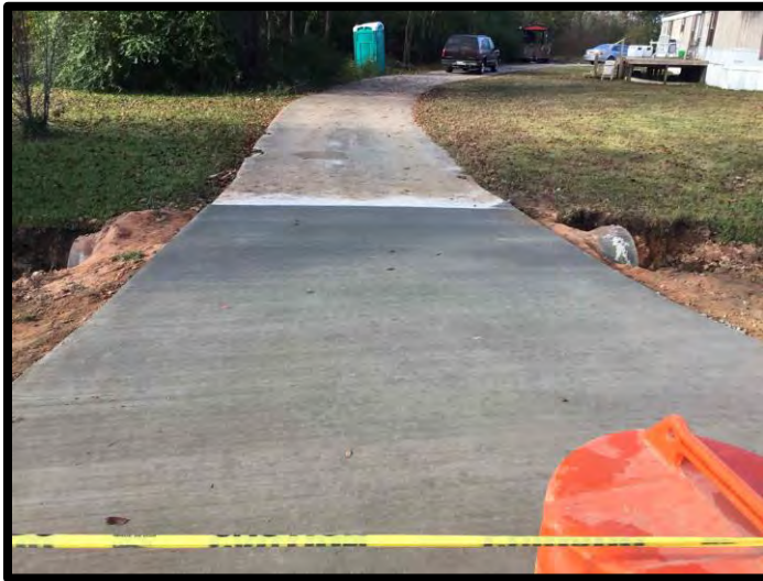
New culvert &amp; driveway repair along MLK Drive
