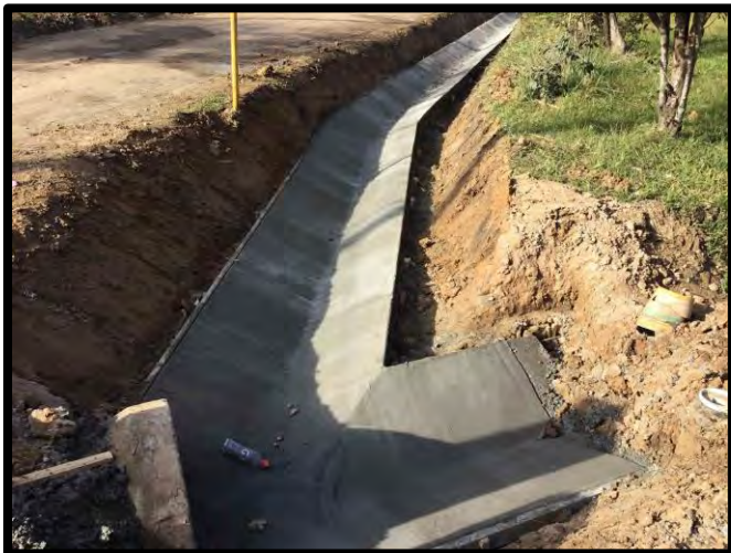
Roadside ditch along MLK Drive
