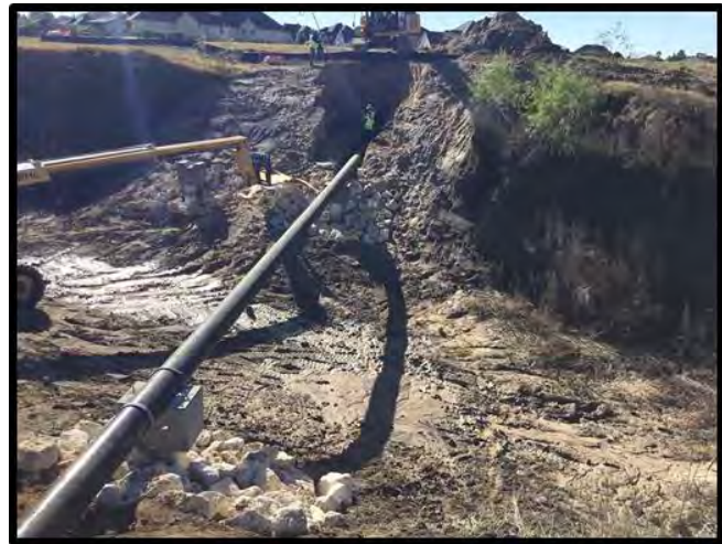
Waterline installed in casing across piles
