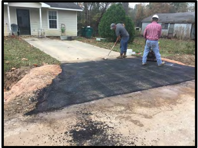
Driveway repair along Baja Road
