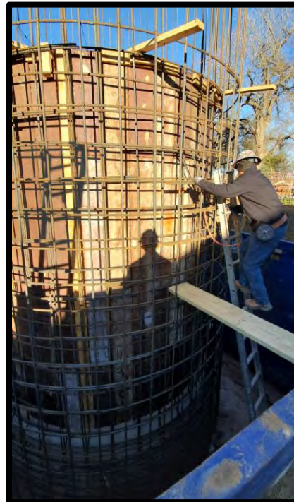
Rebar for new Lift Station No. 1
