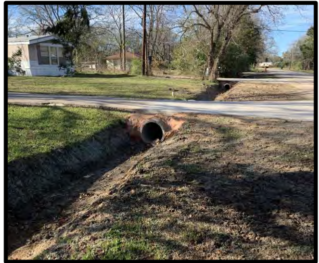
Ditch regrading &amp; new culvert along MLK Drive
