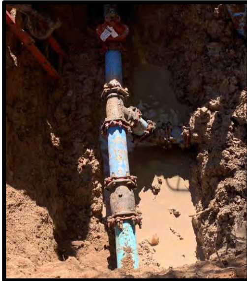
New waterline installed along MLK Drive
