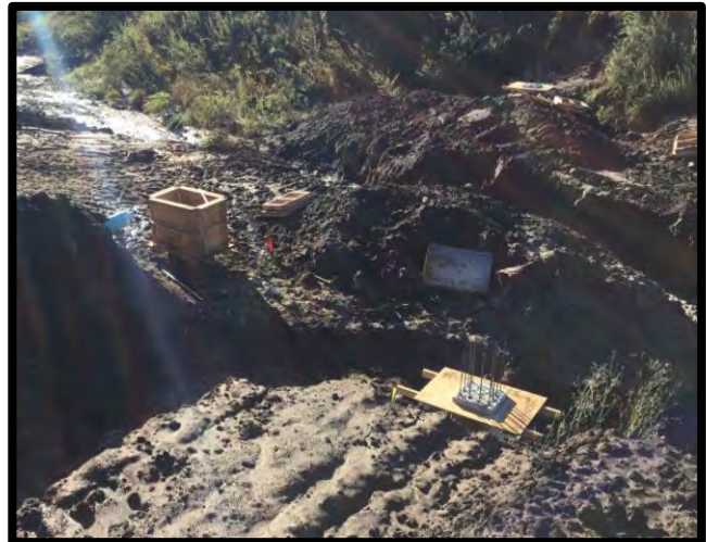
Piles drilled; caps ready to be formed
