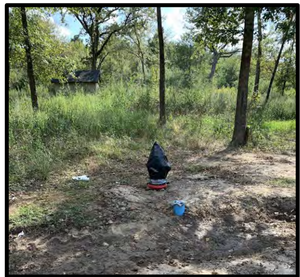
New fire hydrant set along Baja Road
