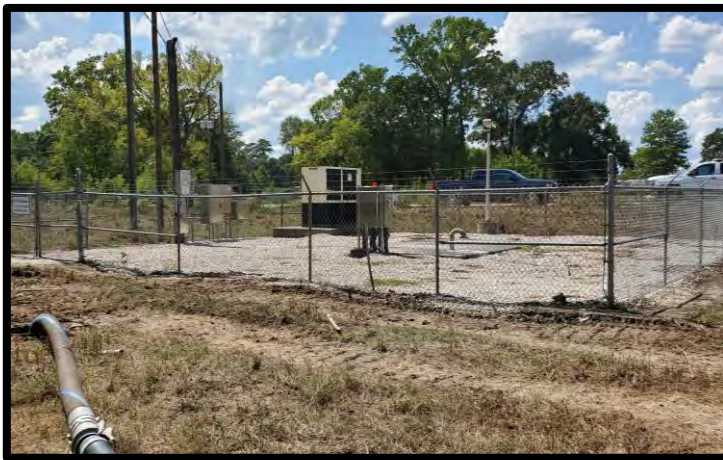
Lift Station No. 1 pre-demolition
