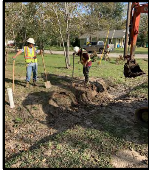
Ditch regrading at MLK Drive &amp; McGinnis
