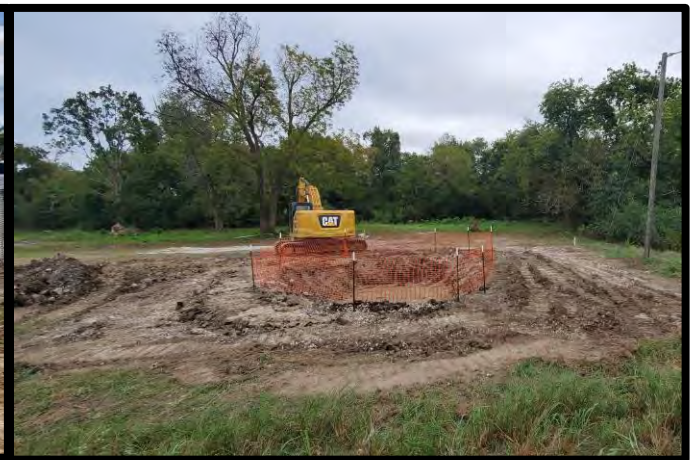
Lift Station No. 1 post-demolition
