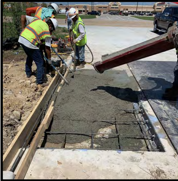
New concrete at driveway after abandoning MH
