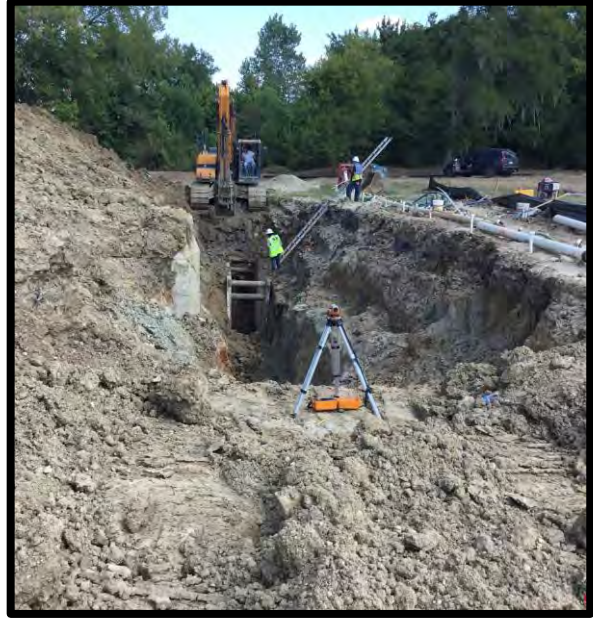
Connection to Phase I sanitary sewer line
