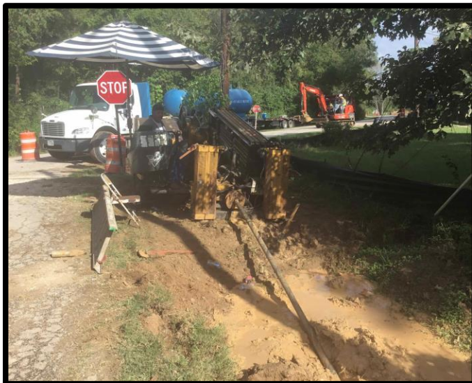
Contractor boring along Baja Road
