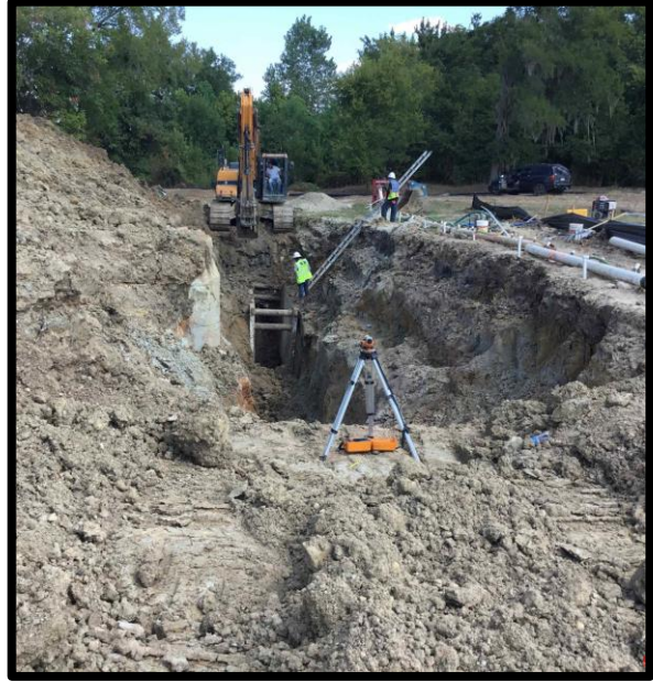
Connection to Phase I sanitary sewer line
