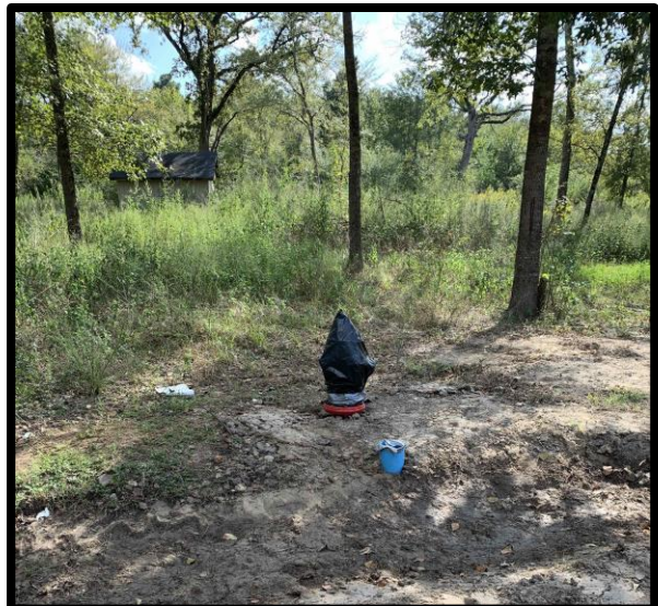
New fire hydrant set along Baja Road
