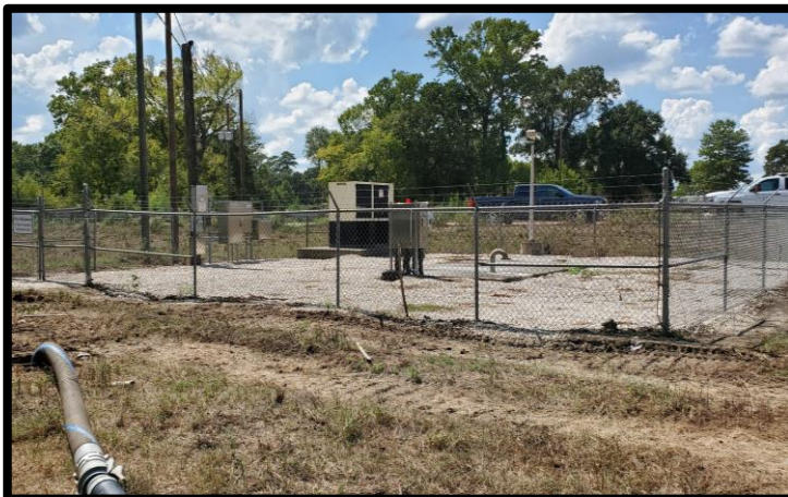
Lift Station No. 1 pre-demolition
