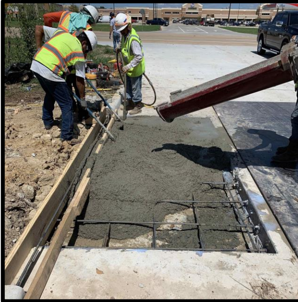
New concrete at driveway after abandoning MH
