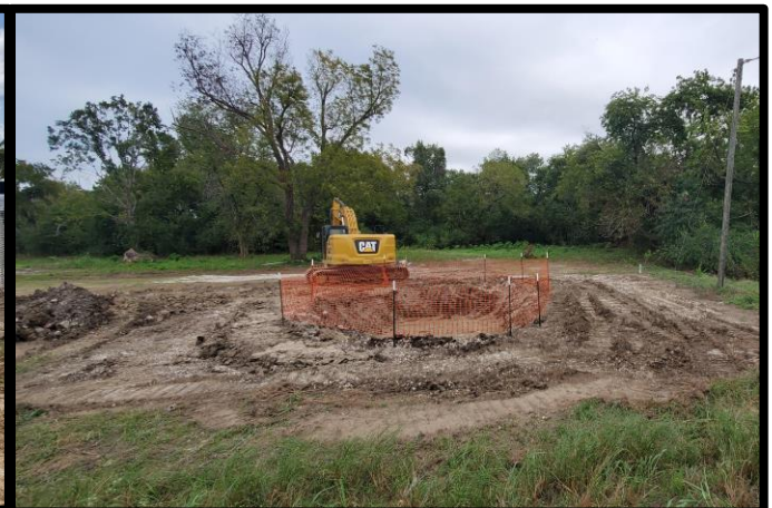
Lift Station No. 1 post-demolition
