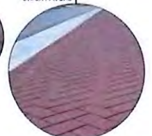
CROSSWALK BRICK PAVERS
