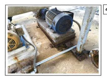
Findings: Motor and motor skid are corroded.
