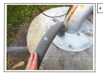
Findings: The flexible conduit is failing.
