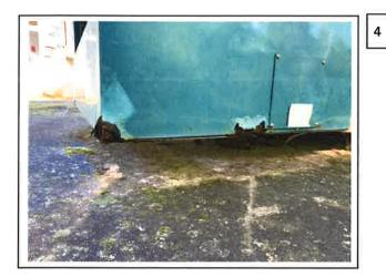
Findings: Generator enclosure is corroding.
