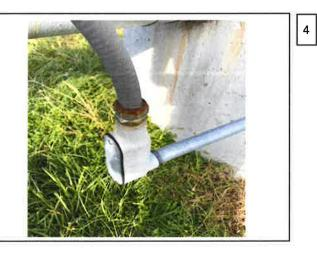
Findings: Myers hubs are corroded.
