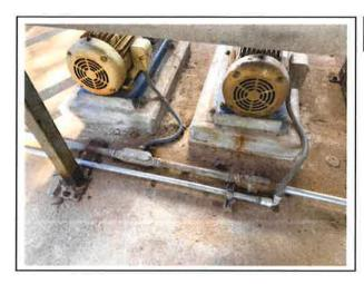
Findings: Conduit and hardware are corroded.
