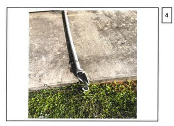
$\underline{\text{Findings}}$ : The conduit for generator ground is broken.
