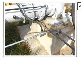
Findings: Myers hubs are corroded.
