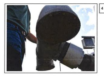
Findings: The well vent insect screen is damaged.
