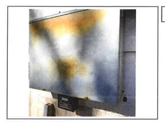
Findings: Junction box is corroded.
