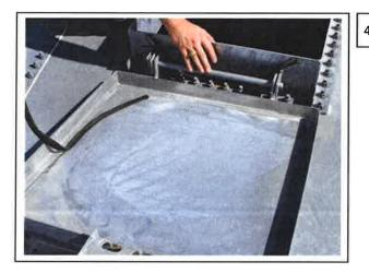
Findings: The gasket on the access hatch is missing.
